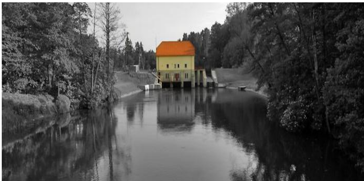
Hydro power plant Łyna
