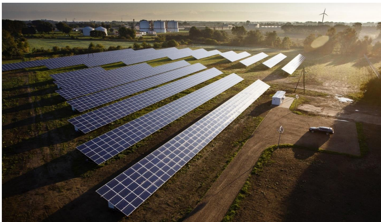
Photovoltaic farm in Bystra
