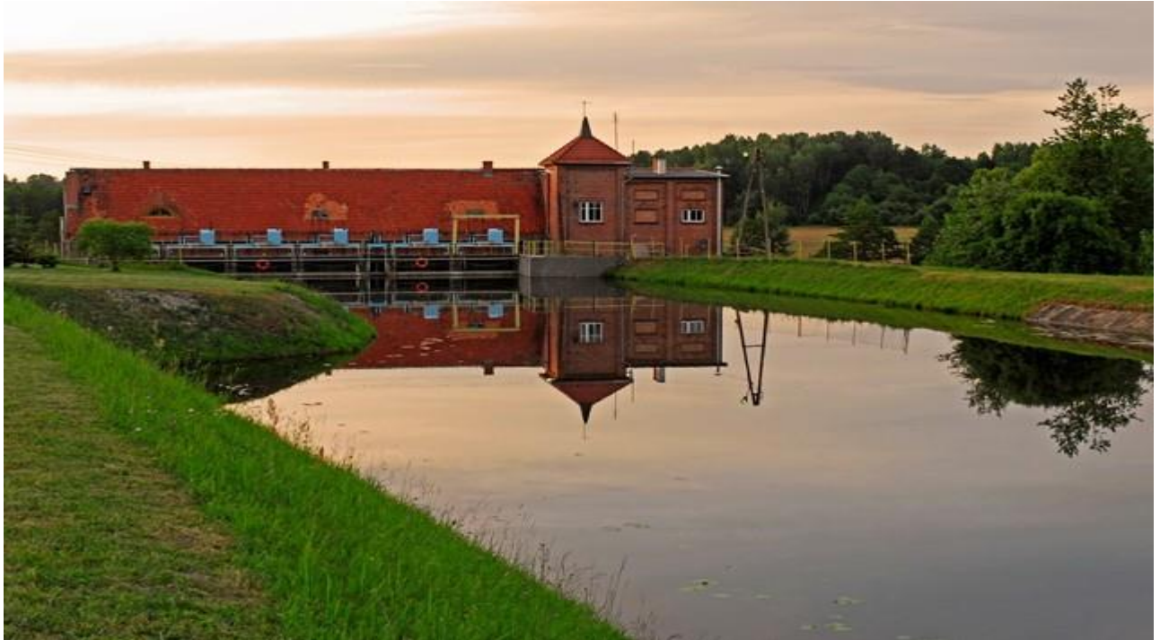
Hydro plant in Pierzchały
