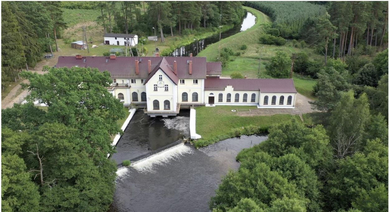
Hydro plant in Żelkowo
