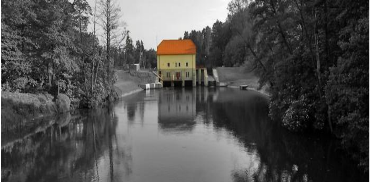
Hydro power plant in Łyna
