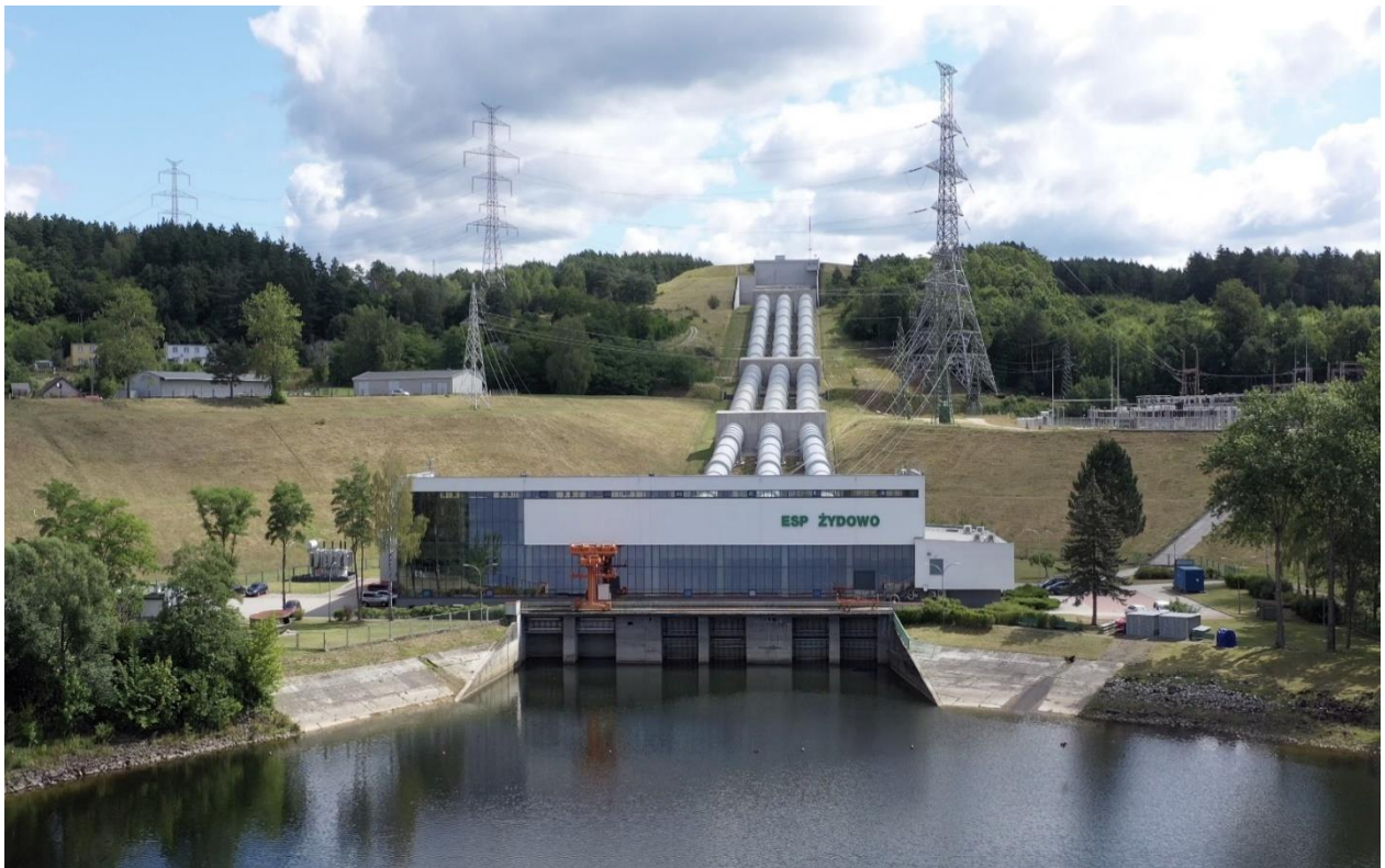
Pumped storage power plant in Żydowo
