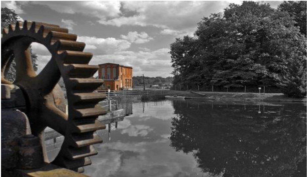
Hydro power plant in Owidz, on the Wierzyce river
