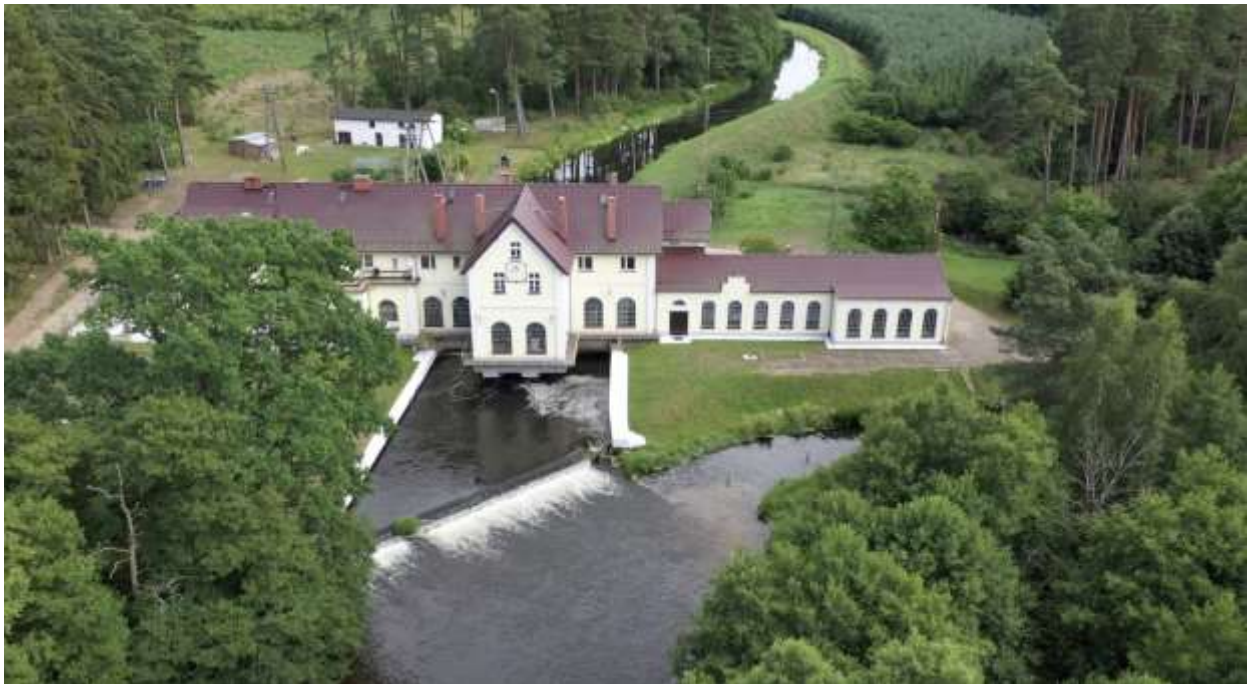
Hydro power plant Żelkowo
