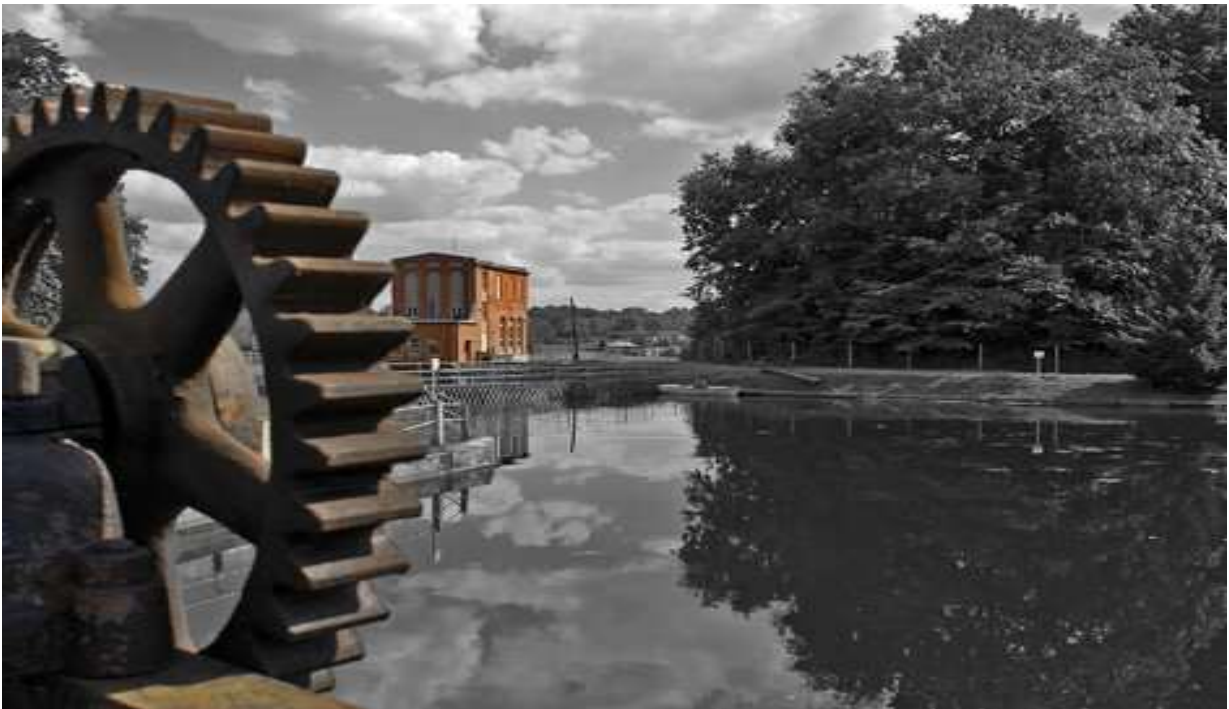
Hydro power plant Owidz, on the Wierzyca river
