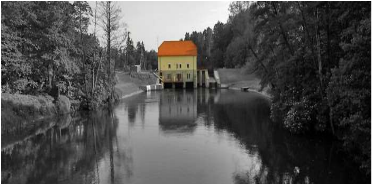
Hydro power plant Łyna
