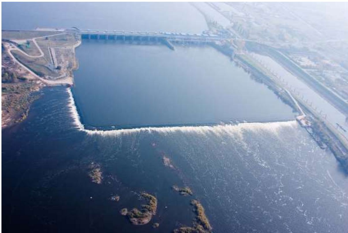
Włocławek Hydroelectric Power Station
