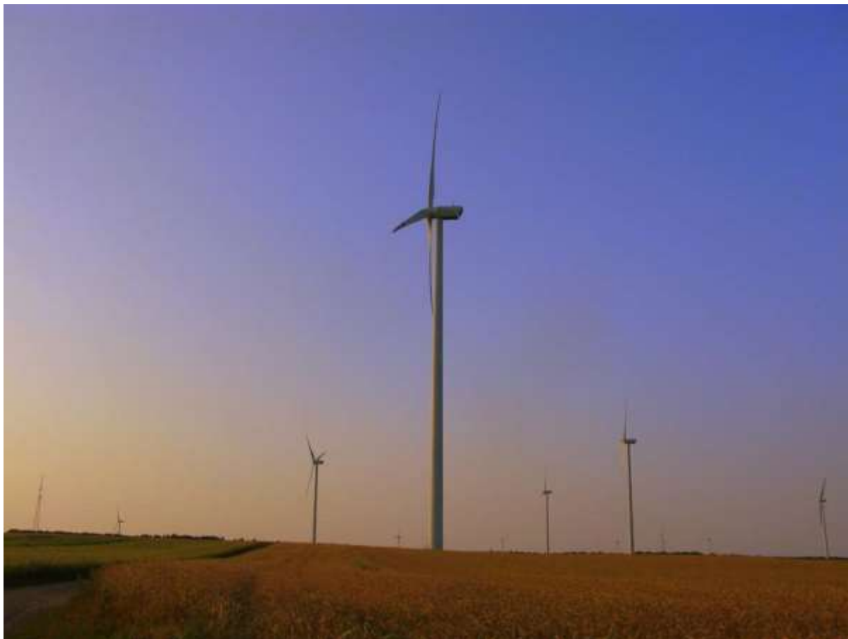
Energa's Wind Farm
