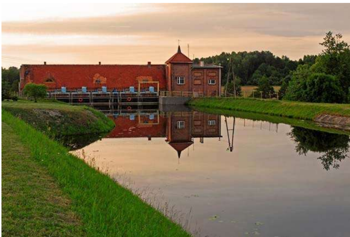
Hydro plant in Pierzchały
