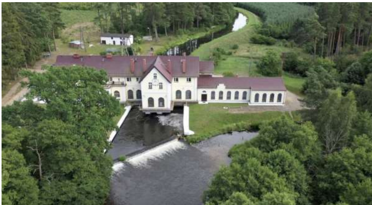
Hydro plant Żelkowo
