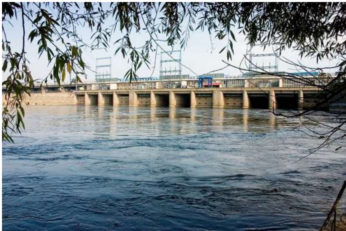
Włocławek Hydroelectric Power Station
