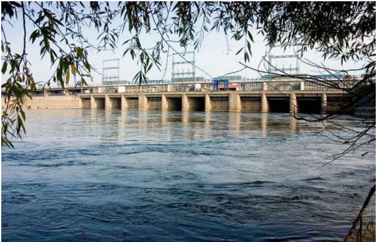
Włocławek Hydroelectric Power Station
