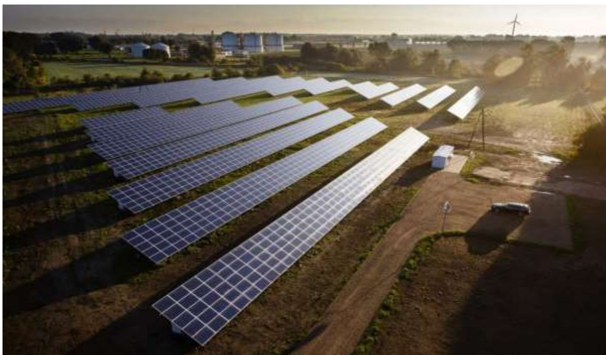
Photovoltaic farm in Bystra
