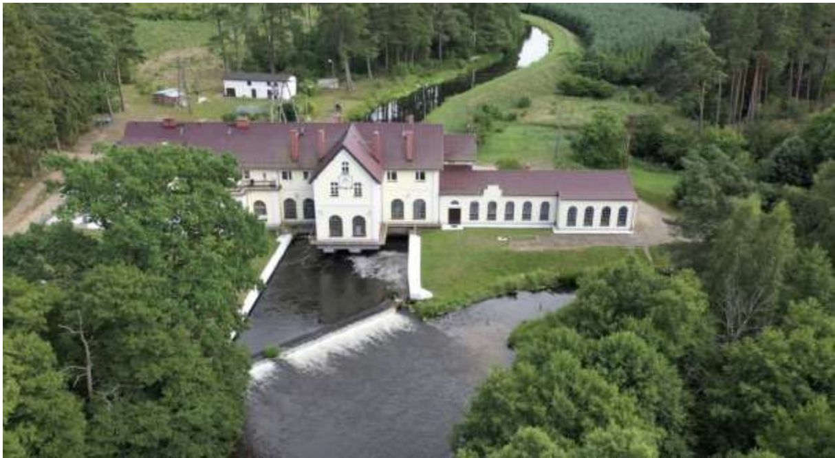
Hydro plant Żelkowo
