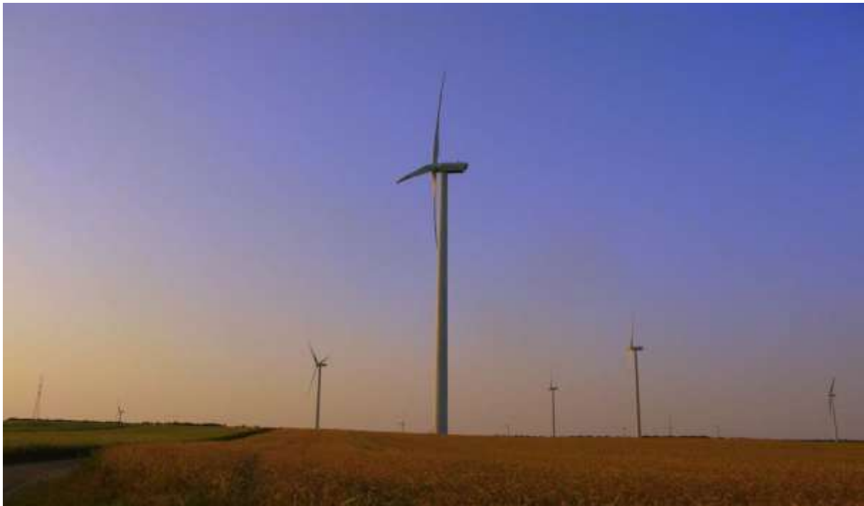
Energa's Wind Farm
