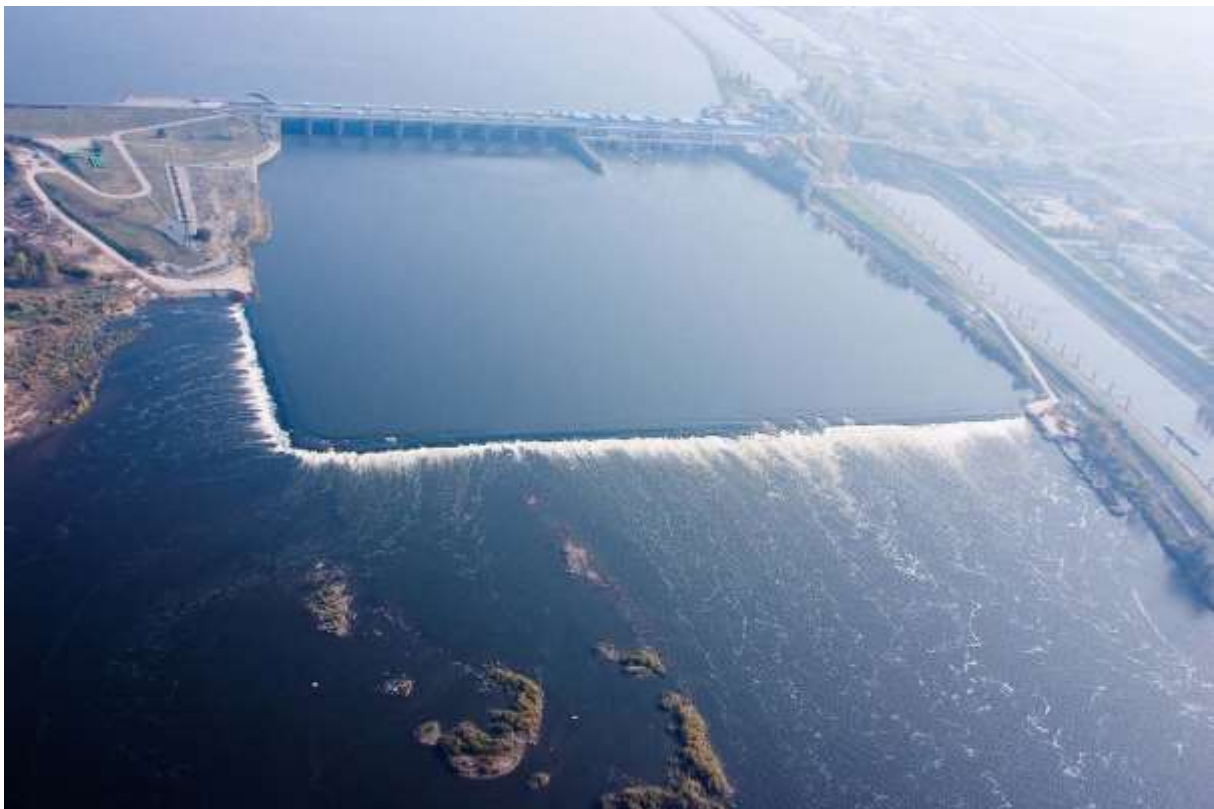
Włocławek Hydroelectric Power Station
