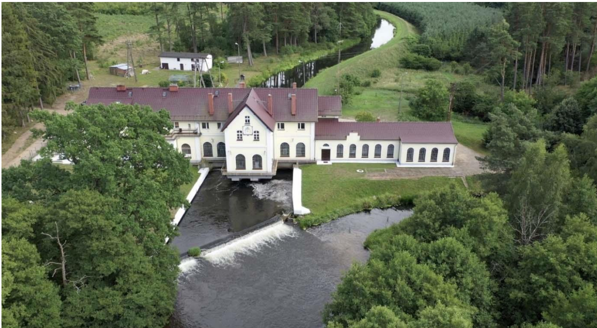
Żelkowo hydro plant
