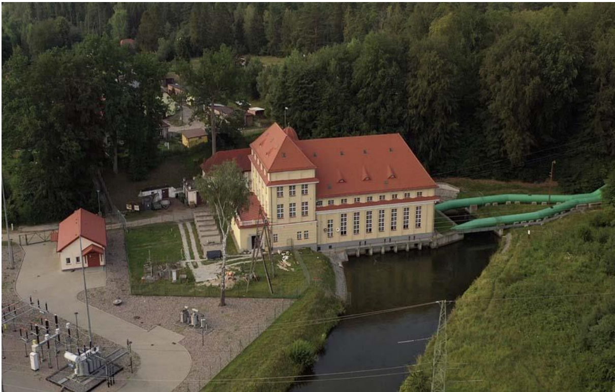
Water power station in Gałężnia Mała on river Stupia
