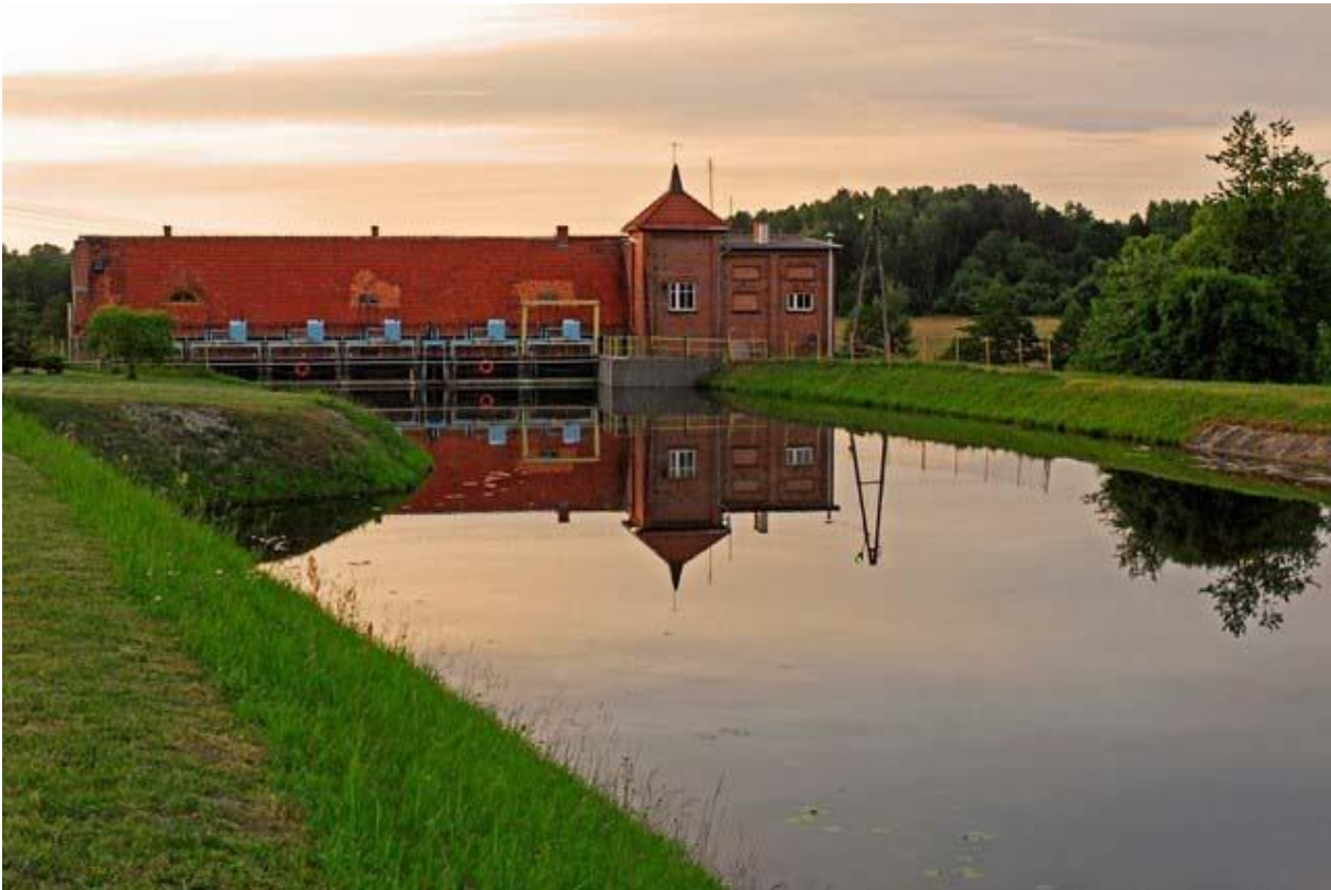
Pierzchały Hydroelectric Power Station
