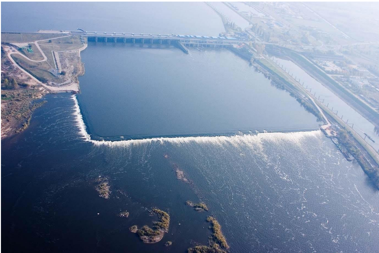
Włocławek Hydroelectric Power Station
