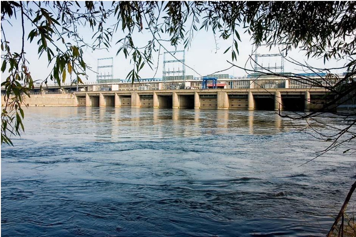
Włocławek Hydroelectric Power Station
