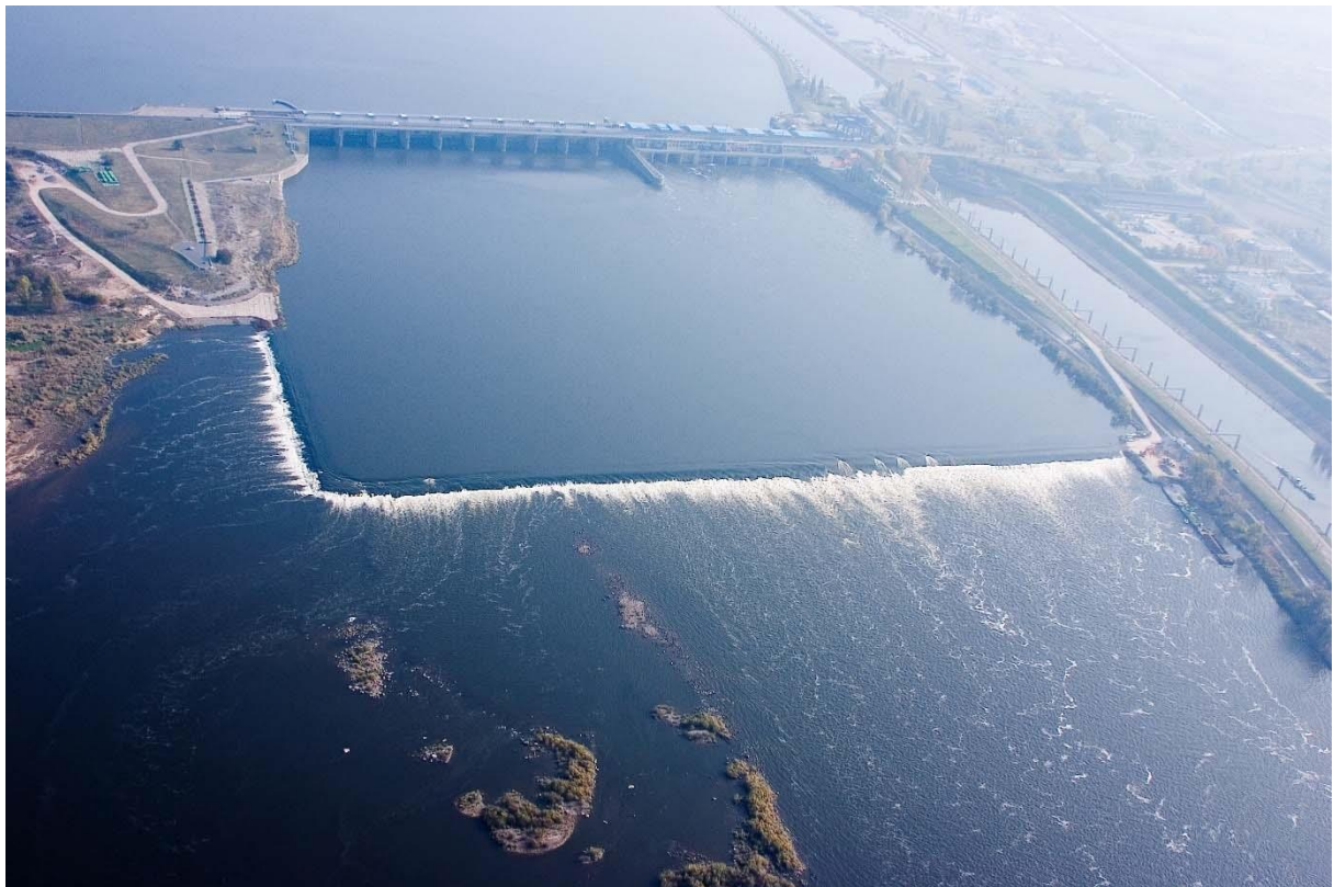
Włocławek Hydroelectric Power Station
