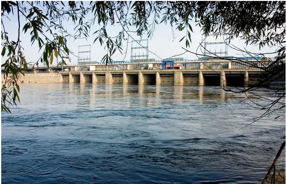
Włocławek Hydroelectric Power Station
