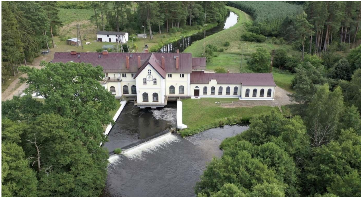
Hydro plant Żelkowo
