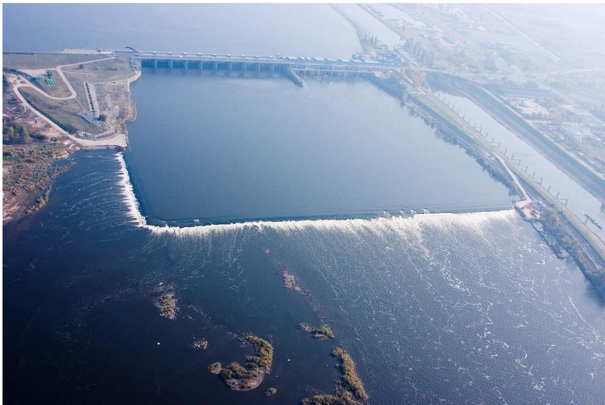
Włocławek Hydroelectric Power Station
