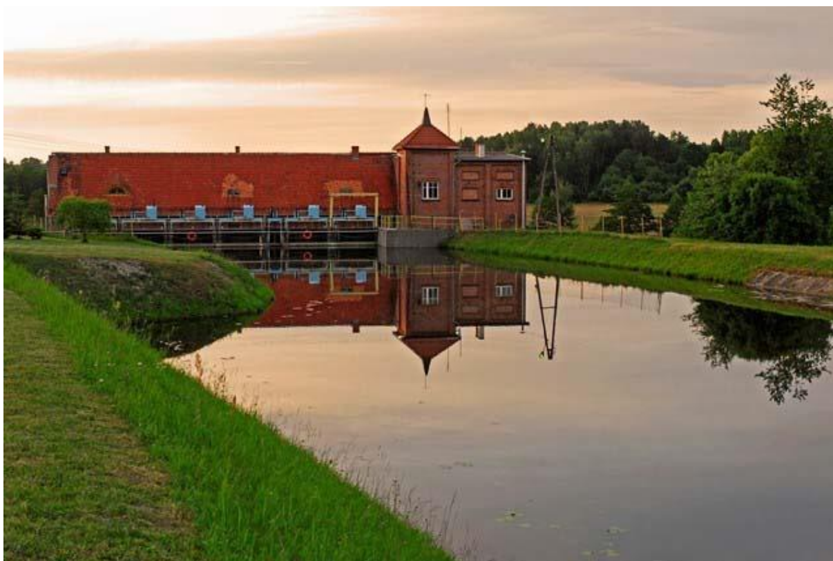
Hydro plant in Pierzchały
